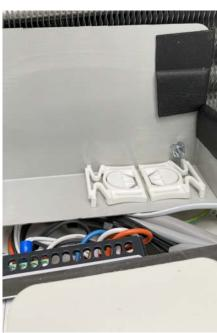
On either side of the controller you will see 2 white fixing clips. Push the white tabs of these clips slightly inwards to the controller. This will unlatch the tabs of the white clips and allow you to slide the clips off the back of the controller.
