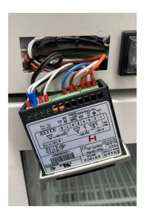
Once the white clips have been removed you can then push the controller through the front of the fridge so you can access the wires. Using a small flat head screw driver, unscrew each of the wires from controller.
