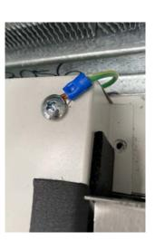
To remove this plate to be able to access the controller, undo the screws on either side of the plate. You DO NOT need to unscrew the green earth wire on the back of the plate.
