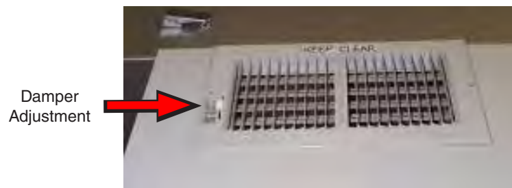
Figure 6.4b: Damper adjustment location at top rear of chiller.
