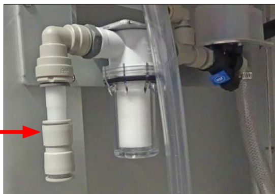
Figure 6.4g: Tube adapter for 12 mm water supply tube.
